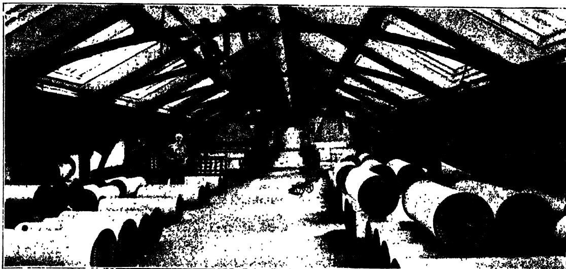
SIZING ROOM (MESSRS. HORROCKSES, CREWDSON AND CO., LTD.).
